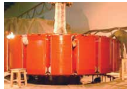
144MW KGA-HEP: Electrical Equipment Rotor being assembled
