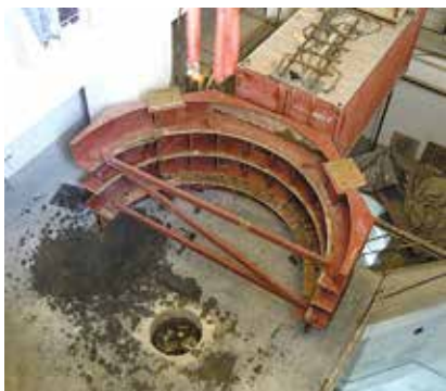
Preassembling Stator Frame
