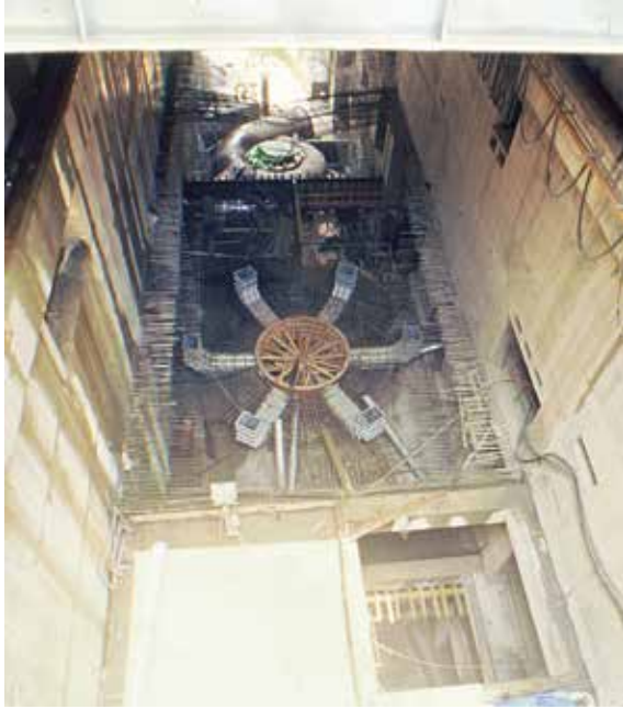
Installations for embedding turbines
