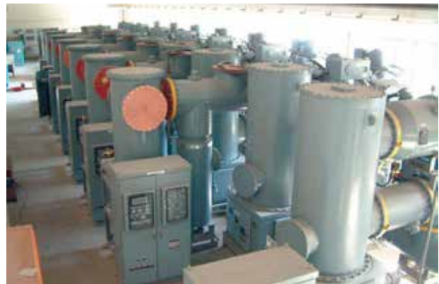
132kV GIS Switchgear at KGA-HEP
