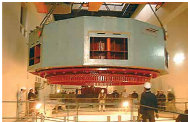
Electrical Equipment: KGA-HEP Generator Stator being shifted to Pit
