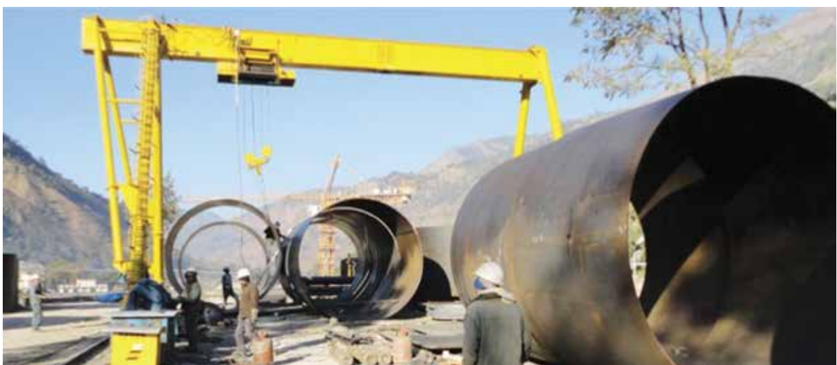
Hydromechanical Equipment - Penstock Steel Liner, 30 MW Chameliya HEP
