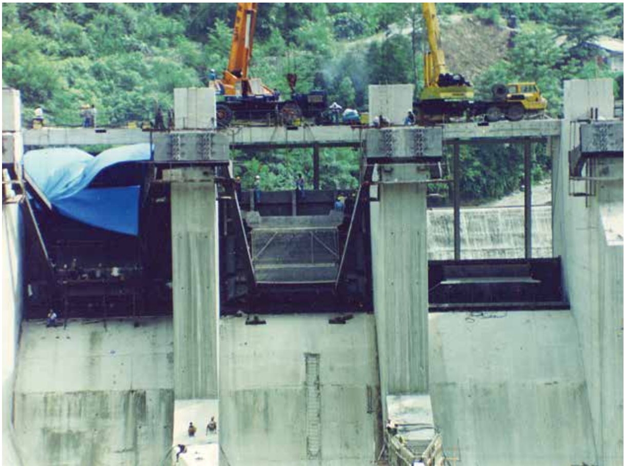
Hydraulic Steel Structures and Systems for 144MW Kali Gandaki A Hydroelectric Project. Above photos show various stages of construction.
