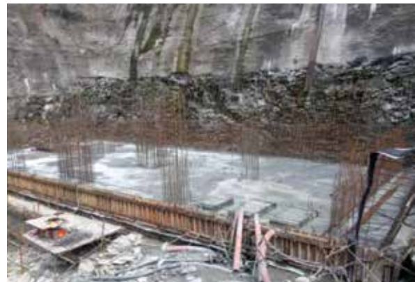
Raft Concrete Works in Auxiliary Powerhouse
