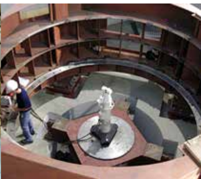
Dovetail Bar installation
