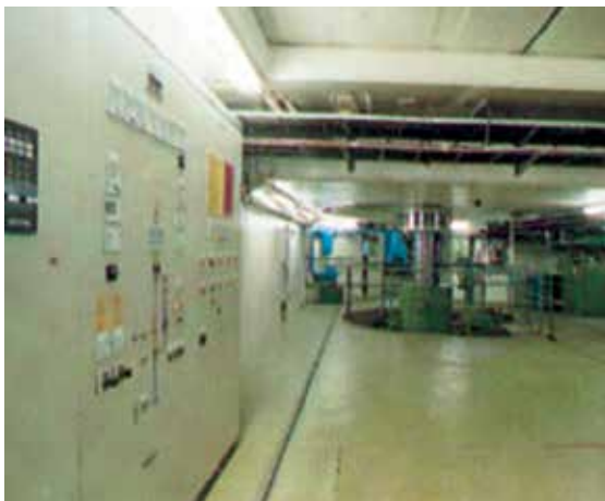
Control Panel at 69MW Lower MHEP
