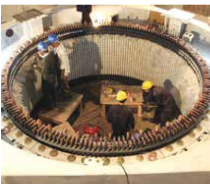
Stator winding work
