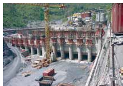
144 MW KGA-HEP: Embedding Hydraulic Steel Structures Steel Gates
