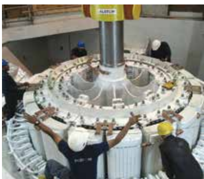
Inserting Rotor
