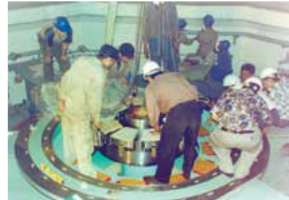
Electrical Equipment Generator assembling at 144 MW KGA-HEP
